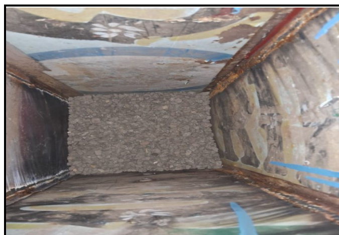
Fig.3: Permeable Layer During Preparation
